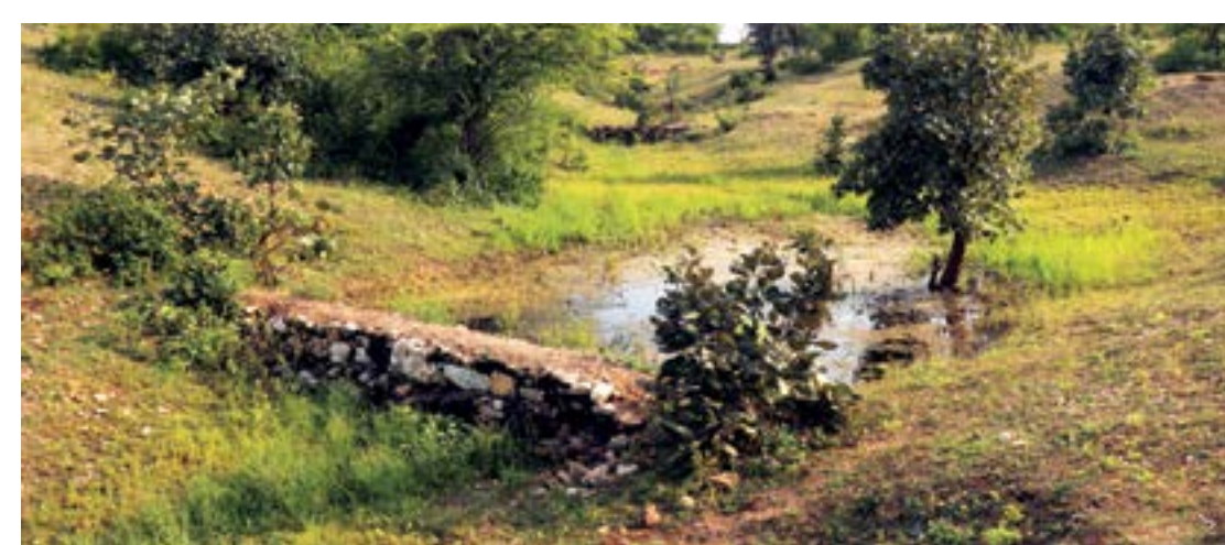
Photo: Gully plugs to treat small water streams.
