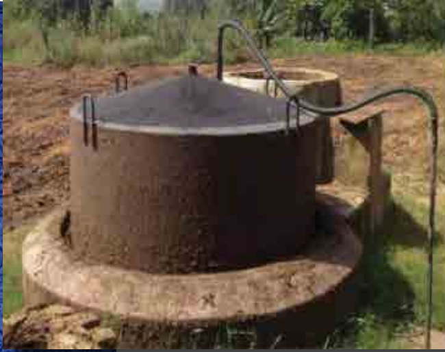
Bio gas plant
